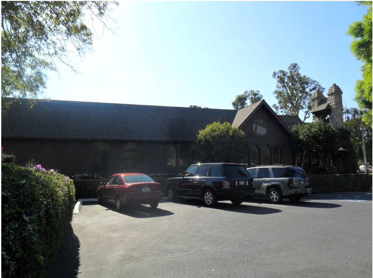
Figure 15 All Saints By-the-Sea Church at 83 Eucalyptus Lane, Montecito North elevation Looking southwest
