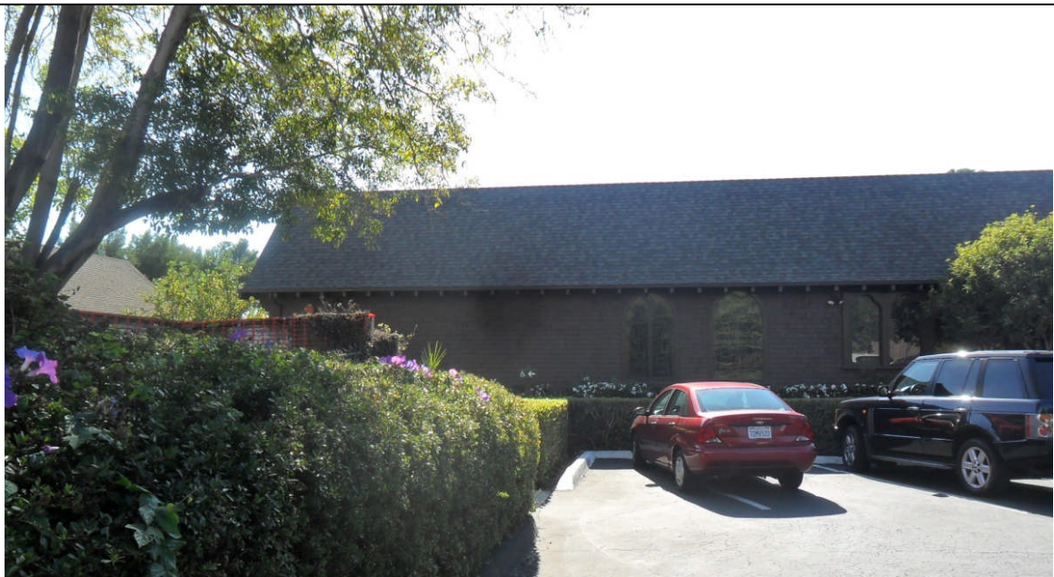
Figure 16 All Saints By-the-Sea Church at 83 Eucalyptus Lane, Montecito North elevation Looking south
